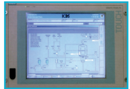
OP or PC: SIEMENS or ALLEN-BRADLEY SCADA SYSTEM DESIGNED FOR FDA 21 CFR PART 11
