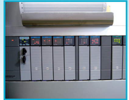
PLC: SIEMENS or ALLEN-BRADLEY
