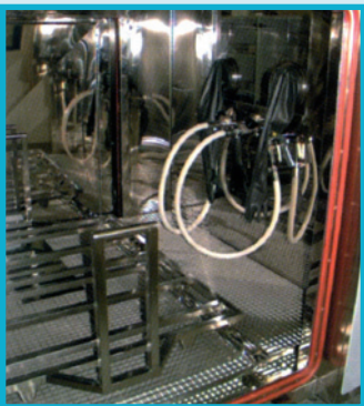
INTERNAL FINISHING OF WASHING CHAMBERS
