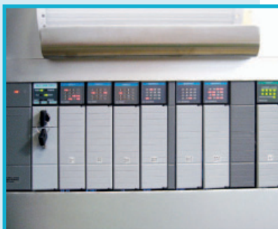
PLC: SIEMENS or ALLEN-BRADLEY
