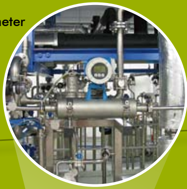
• Block valve technologies
